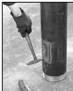
Cut hole with cutting torch; pry out cut portion (shown below).
