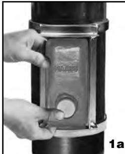
Using cutting guide, establish location of hole to be cut.
