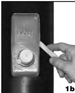
Trace outline of housing onto well casing.
