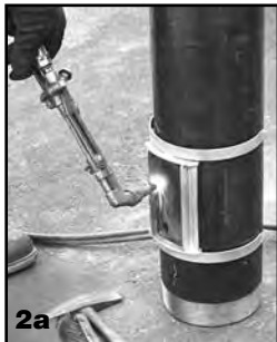
Cut hole with cutting torch; pry out cut portion (shown below).
