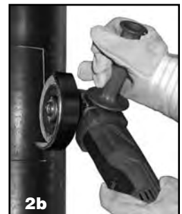
Or use a 4 1/2" hand grinder to cut opening.
